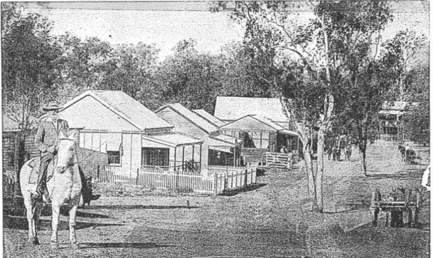
SAPPHIRE TOWN MAIN STREET LOOKING EAST The buildings faced Retreat Creek (right of picture)
